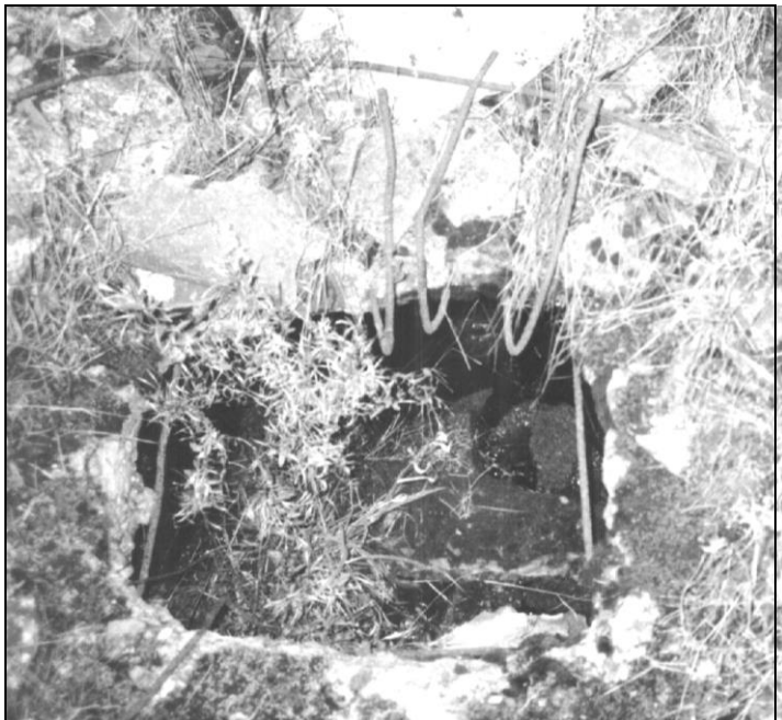
III. 25: Concrete roof of Morgue 1 of Crematorium II in Birkenau. Provan's opening 7 in October 1991. © Carlo Mattogno
