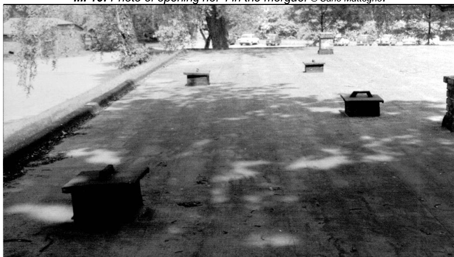
III. 11: Photo of the roof of the morgue. All four shafts constructed by the Poles after the war. © Carlo Mattogno.
