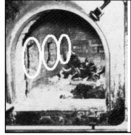
III. 2: Openings in walls of center muffle of Buchenwald triple-muffle furnace (=Birkenau furnaces, highlighted with white ellipses). 10
