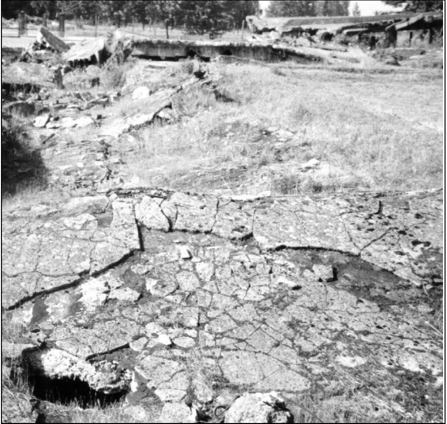
III. 6: The reinforced concrete roof of Morgue 1 of Crematorium II in Birkenau in August 2000. © Carlo Mattogno
