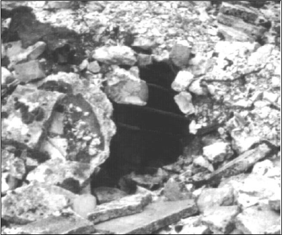
III. 32: Concrete roof of Morgue 1 of Crematorium II in Birkenau. Provan's opening no. 8 in August 2000. © Carlo Mattogno
