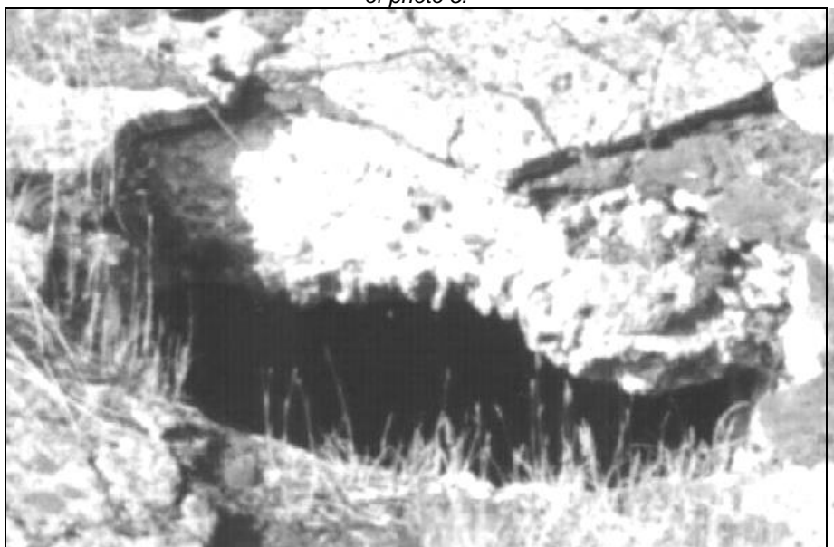
III. 20: Concrete roof of Morgue 1 of Crematorium II in Birkenau. Provan's opening 2 in July 1992. © Carlo Mattogno
