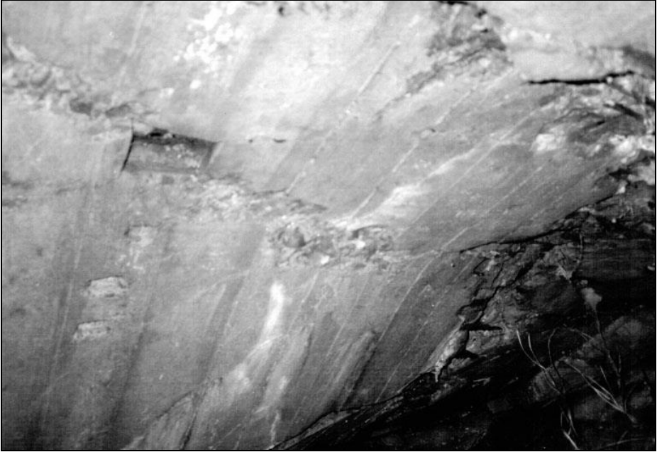
III. 11: Recess in the concrete ceiling of Morgue 1 of Crematorium II at Birkenau for a supporting block for the lamps. July 1992. © Carlo Mattogno.
