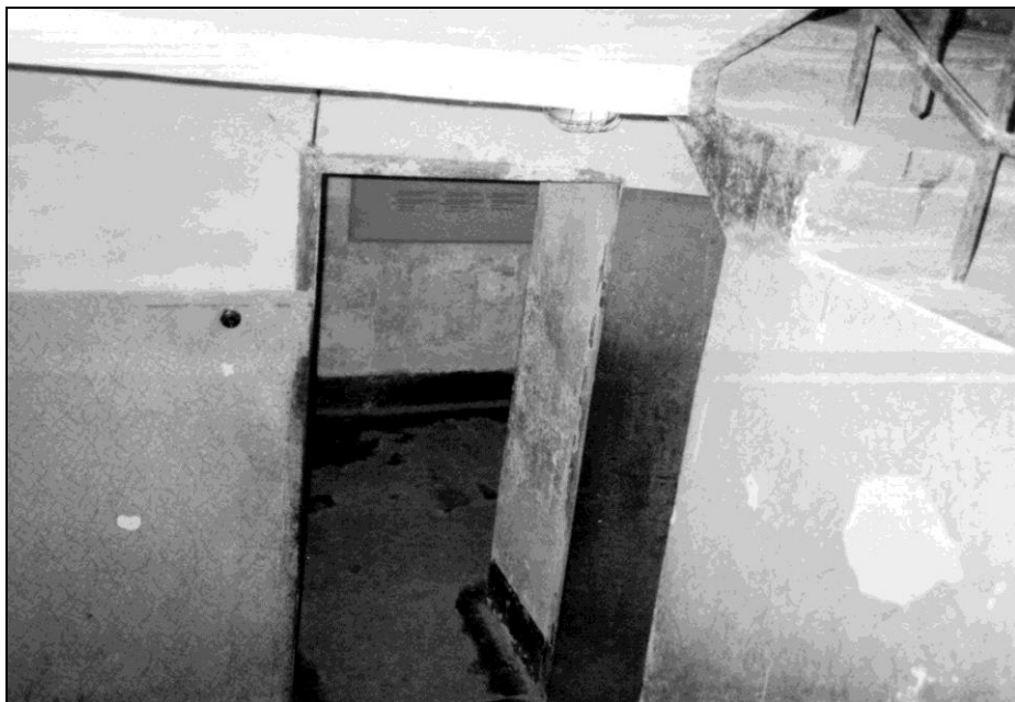
Photo 11: Block 11, inside, steel door of the bunker seen from the stairs.
