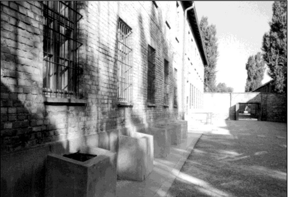
Photo 22: Block 11, outside, wall facing NNE, concrete screens around the window wells of the bunker cells.
