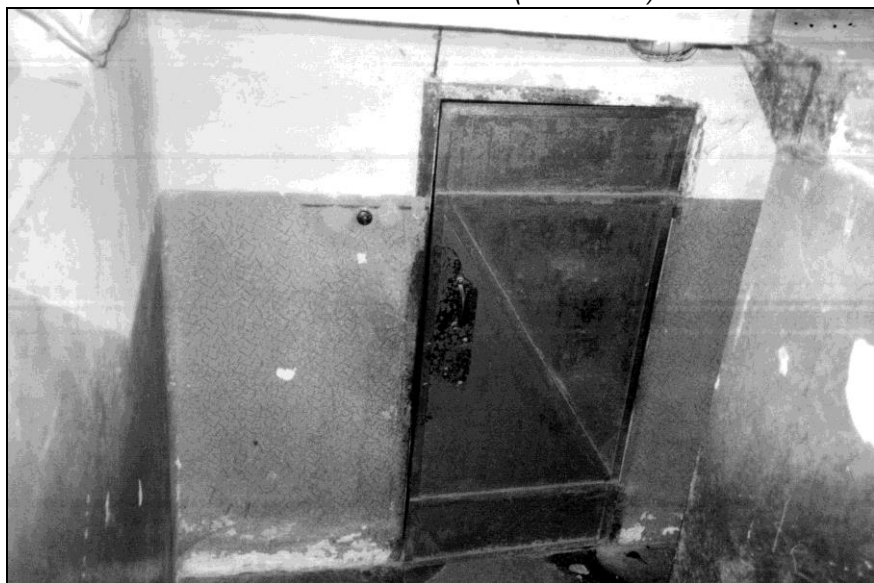
Photo 9: Block 11, inside, steel door of the bunker seen from the stairs.
