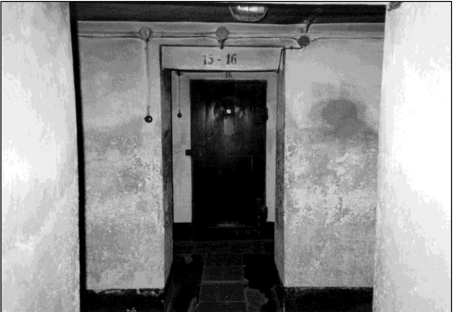
Photo 19: Block 11, inside, bunker, right side, door to cell no. 16.
