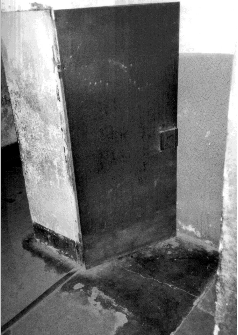
Photo 10: Block 11, inside, steel door of the bunker seen from the stairs.
