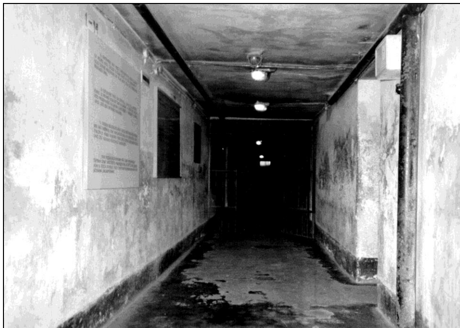
Photo 14: Block 11, inside, bunker, right side, central hallway.
