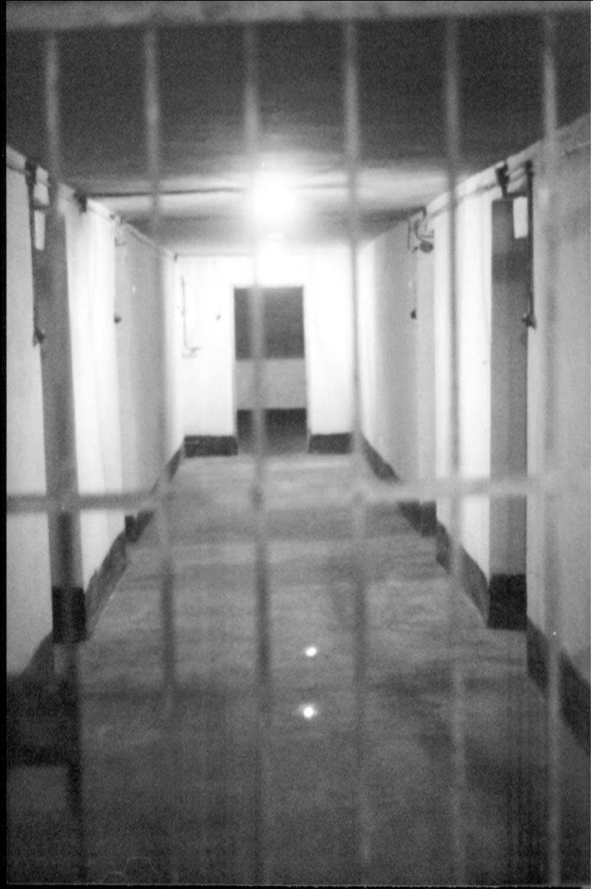
Photo 13: Block 11, inside, bunker, left side, central hallway.
