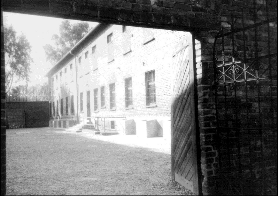
Photo 2: Block 11, outside, wall facing NNE, yard.
