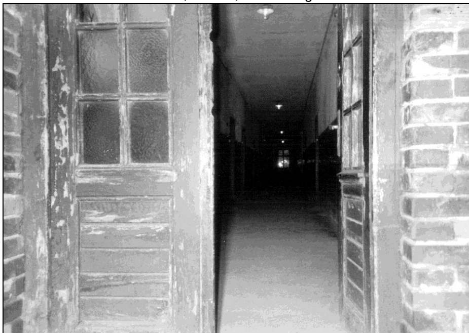
Photo 5: Block 11, outside, wall facing NE, entry door and hallway.
