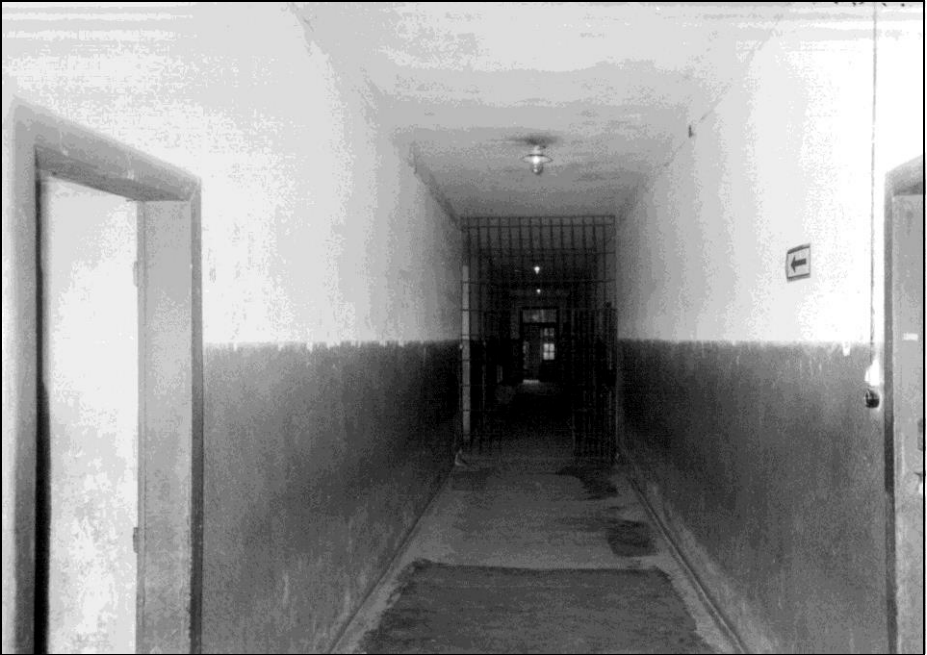
Photo 7: Block 11, inside, ground floor, hallway seen from the opposite side toward the entrance door.
