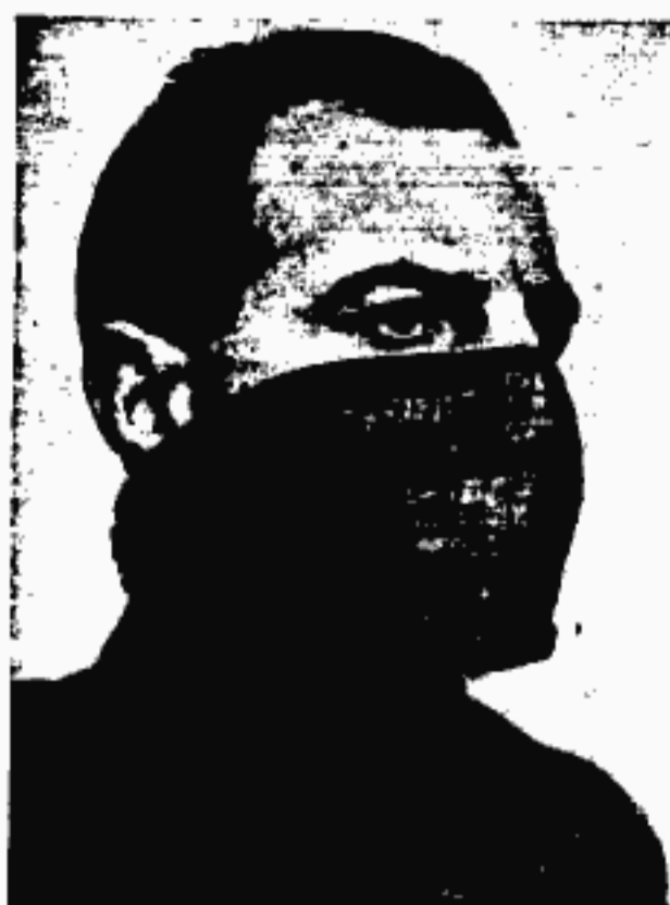
FIG. 108.—First British gas mask, Black Veil Respirator.
