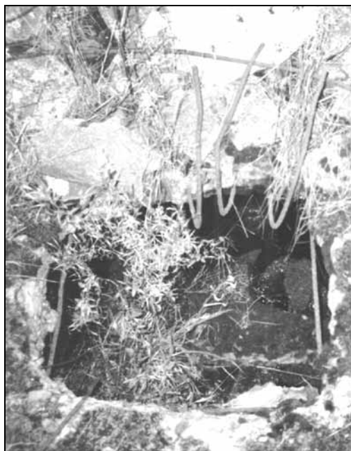
III. 58: Alleged hole for insertion of Zyklon B in roof of morgue #1 (“gas chamber”) of Crematory II. It is clearly visible that it has not been cleared of iron reinforcement bars. They were simply bent backwards. © Carlo Mattogno 1991
