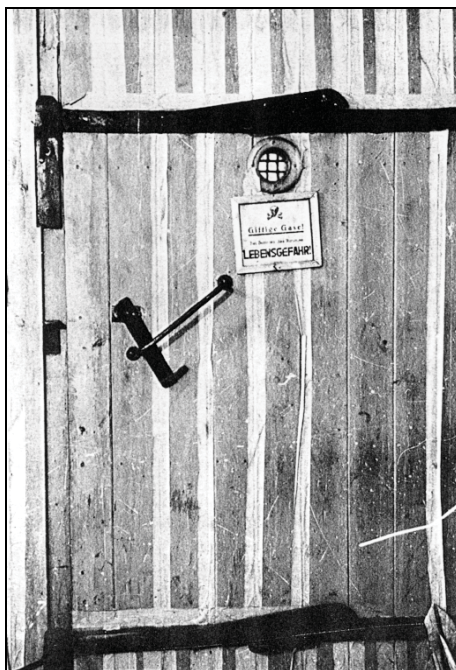
Ill. 79: Makeshift airtight wooden door of a delousing chamber in Auschwitz with peephole and metal grill in front. We are told that this is what airtight doors of homicidal "gas chambers" looked like. Note the flimsy latch!
