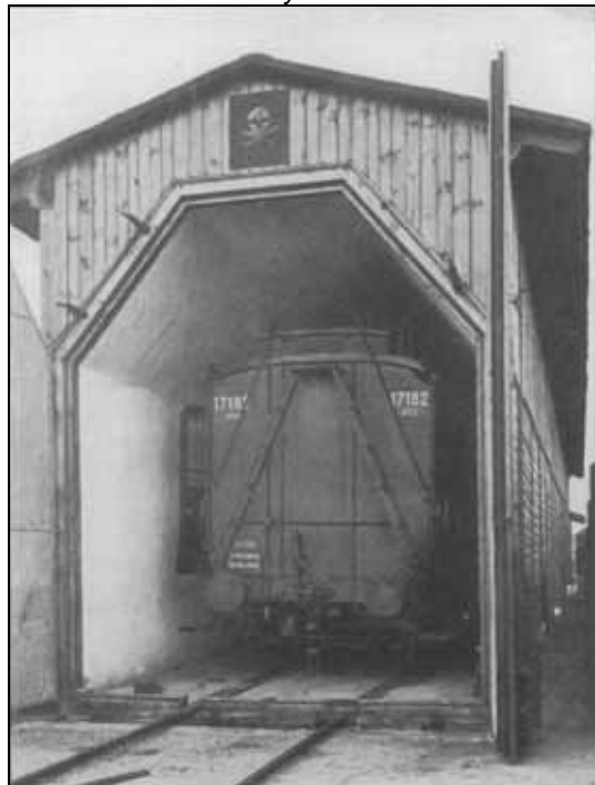
III. 73: A railway cart enters a railway gassing tunnel in Warsaw, Poland (Stock 1924).
