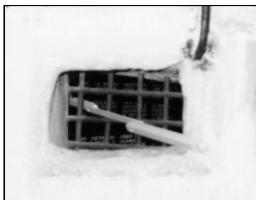
III. 98: Barred opening in the wall of room I in disinestation building 41, Majdanek camp (cf. plan section III. 95) © C. Mattogno
