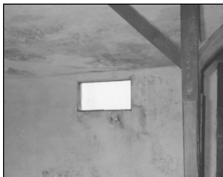
III. 96: Window at the east wall of the chamber IV, barrack 41, (delousing chamber), Majdanek camp (see plan III. 95). © C. Mattogno
