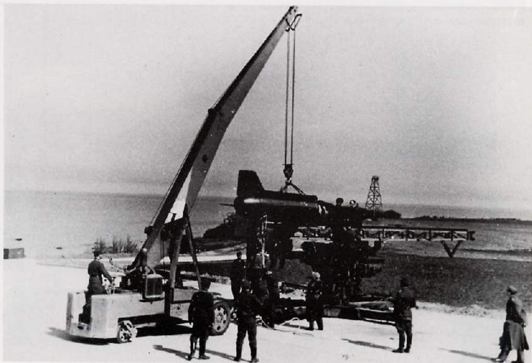
Preparation of an Enzian launcher for a test shot.
